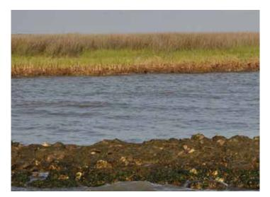
Pictured above is an example of a living shoreline protecting a marsh in the background. With calm, protected waters between the structure and the shore, a diverse habitat is possible for plants and organisms, such as attached animals (like oysters) that provide food for fish and birds.
